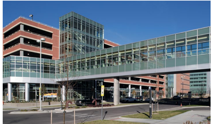
A walkway glazed with Solarban ® 70XL glass connects the medical office building to a 1,500-car garage.
