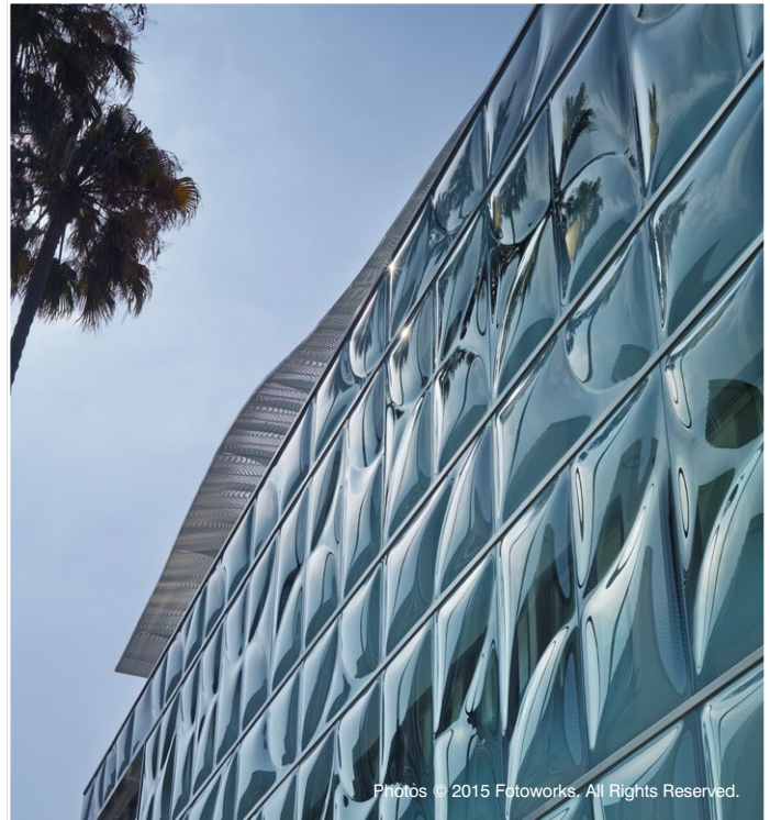
Starphire ® glass by Vitro Glass in combination with carved limestone helped transform a non-descript three-story building into the stunning Gores Group World Headquarters. The façade is composed of three double-paneled, bent-glass patterns with a dozen different custom-printed interlayers sandwiched in between.
