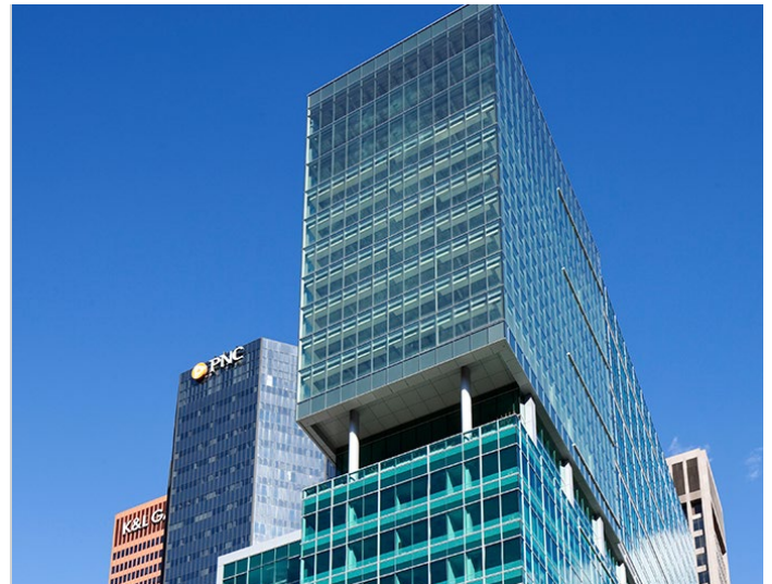
Solarban ® 70XL/ Caribia ® glass casts a soft green tint on the exterior of 23-story Three PNC Plaza.
