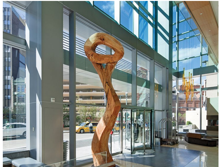
Three PNC Plaza is LEED-certified at the Gold level. The use of Solarban ® 60/clear and Solarban ® 60/ Starphire Ultra-Clear™ glasses provides the interior lobby with high levels of natural daylight while mitigating the effects of solar heat gain.
