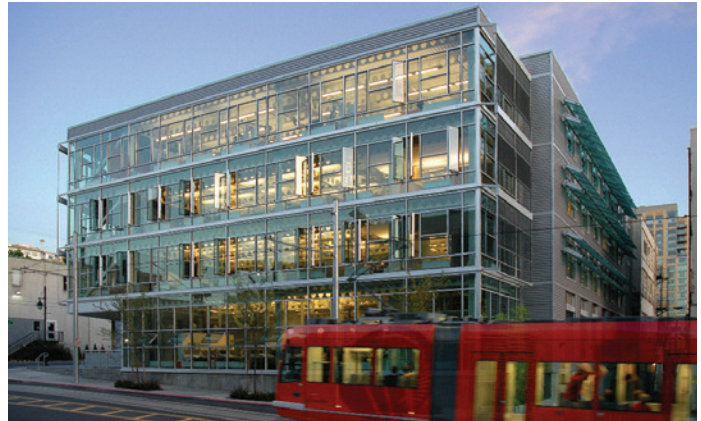
New Solarban 72 Starphire glass is comparable to Solarban 70XL glass, pictured here on AIA COTE award winner, The Terry Thomas in Seattle, with significantly better visible light transmittance and similar solar control.
