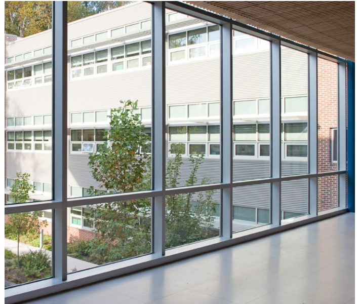
With an overall design concept of bringing the outdoors inside to the students, Solarban ® 70XL glass specified on MPES for its VLT of 64 percent and a SHGC of 0.27.
