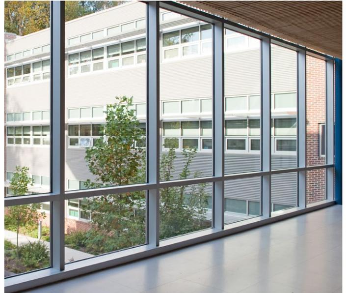
With an overall design concept of bringing the outdoors inside to the students, *Solarban*<sup>®</sup> 70XL glass specified on MPES for its VLT of 64 percent and a SHGC of 0.27.
