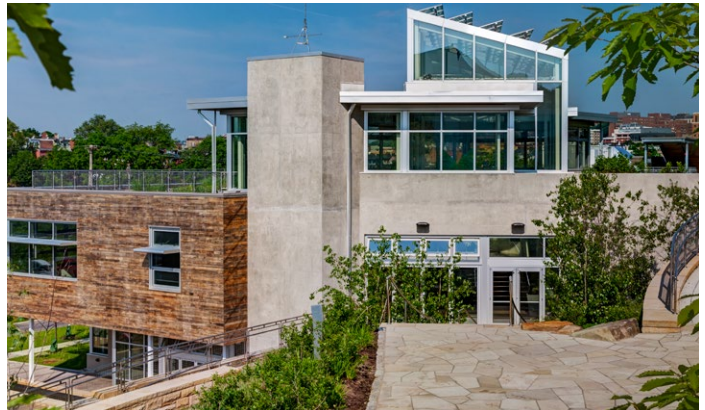
Sungate ® 500/Clear glass combined with Starphire ® and Solarban ® 60/ Starphire ® glasses were specified for the Center for Sustainable Landscapes at Phipps Conservatory and Botanical Gardens, with the goal of satisfying the requirements of the Living Building Challenge. The building is also designed to meet LEED® Platinum certification for sustainable design and SITES certification for landscapes.
