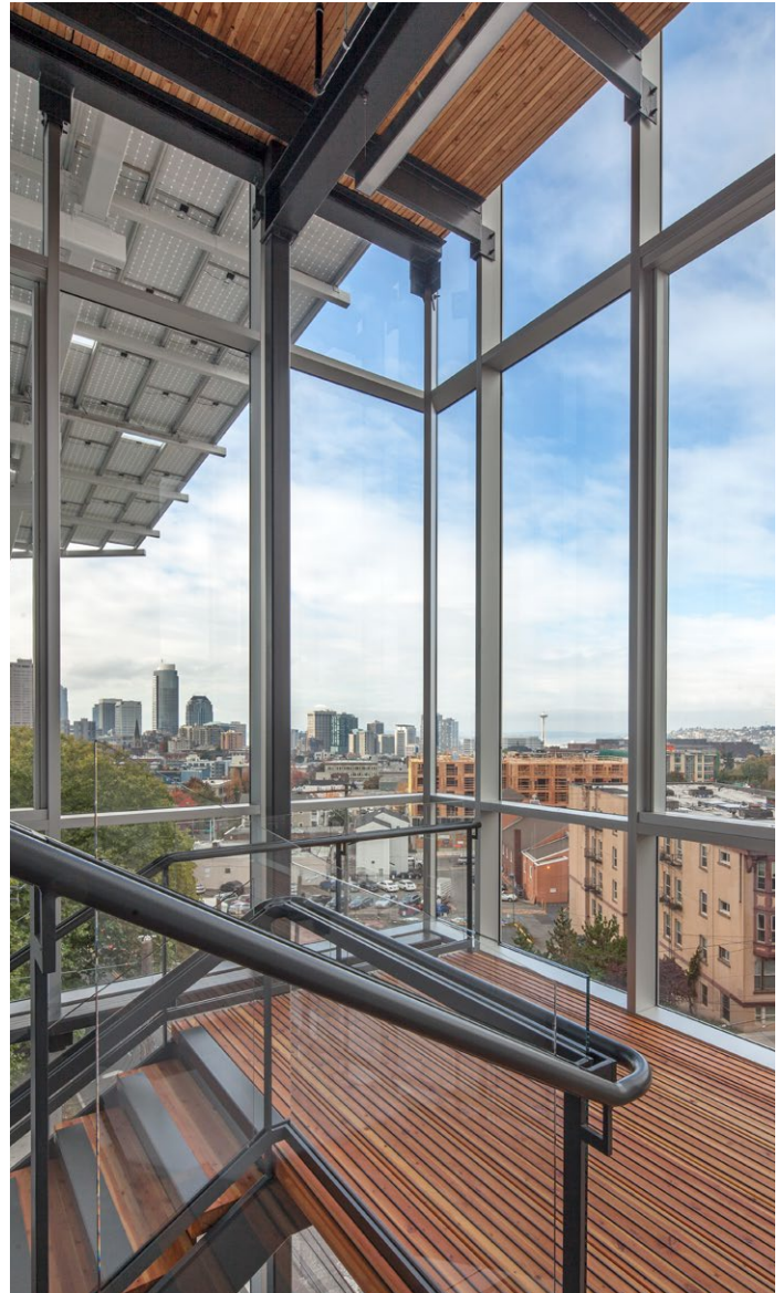
The signature design element of the six-story Bullitt Center in Seattle is the “irresistible stairway,” featuring Starphire ® glass by Vitro Glass, providing panoramic views of Seattle and Puget Sound.
