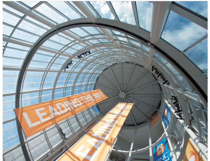
Solarban ® 60 glass by Vitro Architectural Glass transmits light into Prudential Center through two 110-foot-tall glass and steel cylinders.
