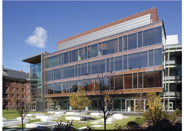
Solarban ® 70XL glass provides maximum daylight and excellent solar control, mitigating the need for artificial lighting and cooling.
