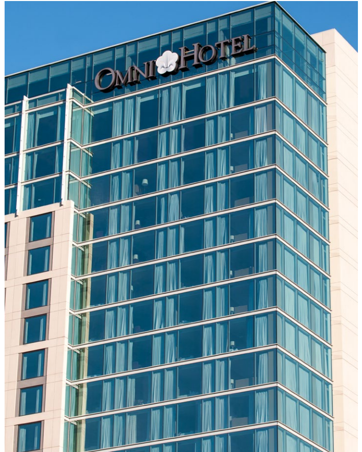
One of the first buildings specified with Solarban ® R100 glass, the Omni Nashville Convention Center Hotel earned LEED® Silver certification from the USGBC.
