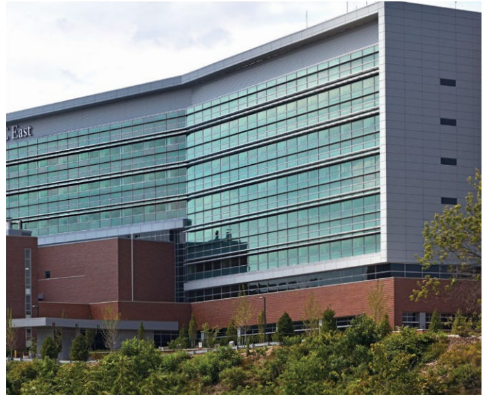
Constructing UPMC East on an east-west axis lowered the hospital’s solar heat gain by 17 percent. Solarban ® 70XL and Solarban ® 60 glasses are part of a super-insulating building envelope that provided the performance and aesthetics the owners desired.
