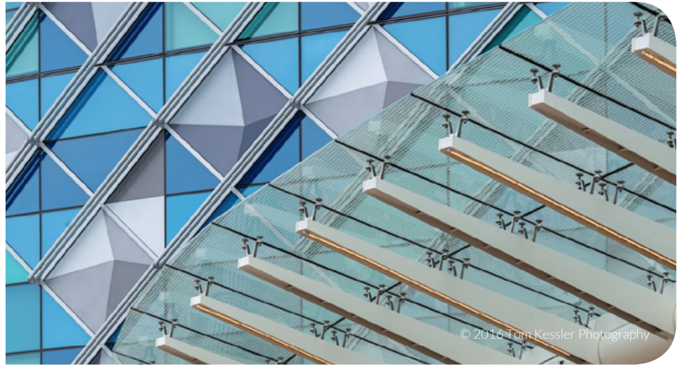
Architects envisioned the signature façade of the hospital to mimic the protective framework of an arbor. The aqua-blue appearance of Azuria ® glass is further enhanced by the application of DURANAR® and DURANAR® SUNSTORM® coatings by PPG.
