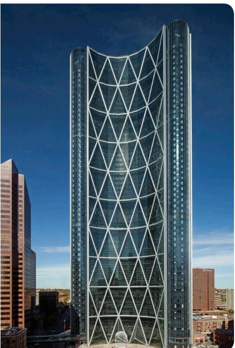
Solarban® z50 glass by Vitro Architectural Glass (formerly PPG glass), shown here on The Bow's distinctive curved shape, provides visible light transmittance (VLT) of 51 percent and a solar heat gain coefficient (SHGC) of 0.31, resulting in a light-to-solar gain (LSG) ratio of 1.64 in a standard, 1-inch insulating glass unit.
