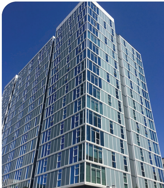
Hoyt Street Yards No. 2 | Portland, Oregon, EUA | Arquitecto: Bora Procesador Certificado Vitro: Vitrum Industries Ltd.
