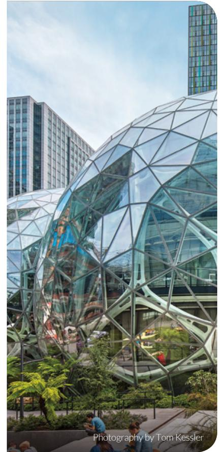
Architects selected *Solarban*® 60 glass on *Starphire Ultra-Clear*® glass after modeling more than two dozen glass products. Because the structure would be housing 40,000 plants, the glass has to be capable of allowing photosynthesis.
