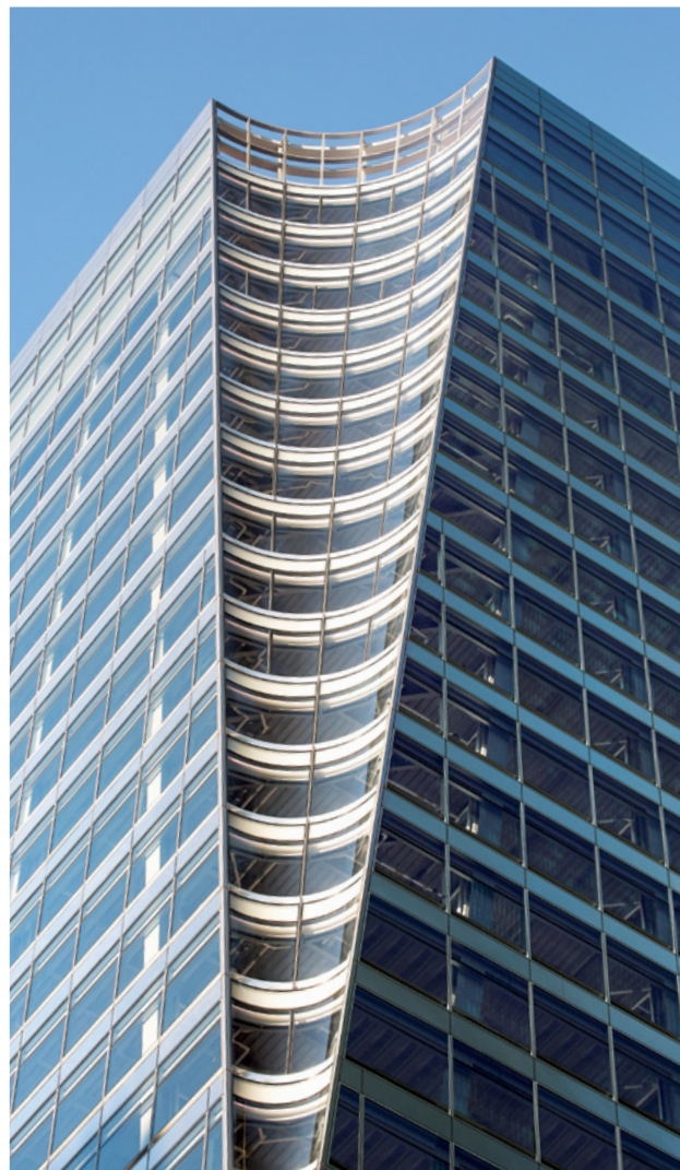
Spandrelite™ glass can be used as a ceramic frit coated glass (like shown) or other spandrel glass materials.
