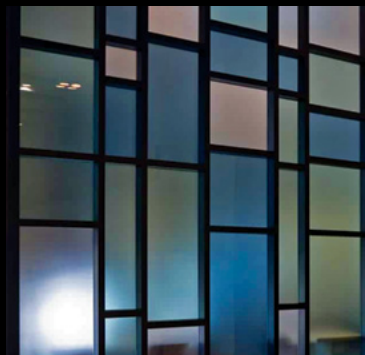
Quebec Civilisation Museum Quebec City, QC, Canada Fabrication by Walker Glass Satin Acid-Etched Tempered Starphire ® Glass
