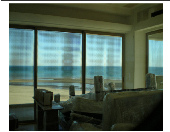
Anisotropy as viewed from inside a condo near a large body of water with ample amount of polarized light. In a different setting and viewing conditions, this strain pattern may not be as noticeable.
